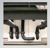
fire rated yet flexible and lightweight elastomeric nitrile rubber material designed for thermal insulation.
